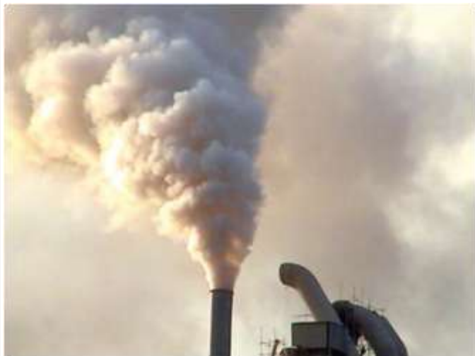
The pollutants released by Hattar Industrial Estate are causing harm to the ecosystem
